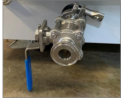
Condenser Drain Port
